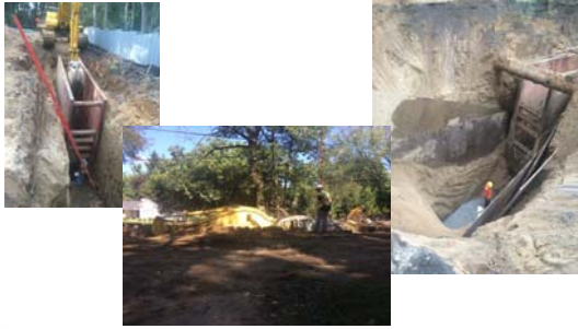
Geddes Ave. Reconstruction
