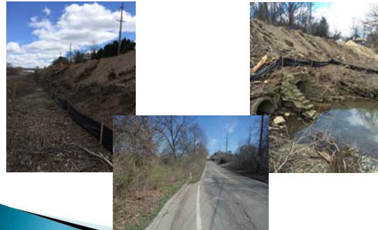
Geddes Ave. Reconstruction
