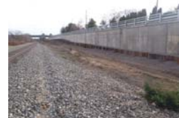
Geddes Ave. Reconstruction
