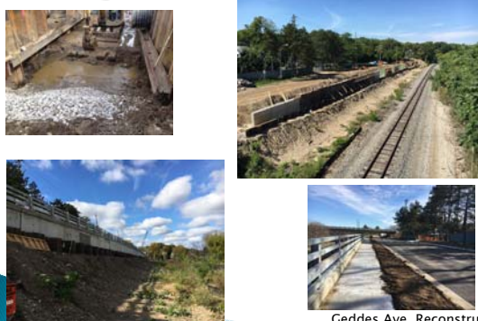
Geddes Ave. Reconstruction
