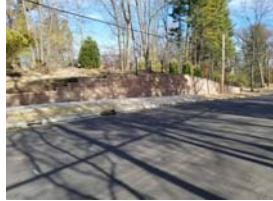
Geddes Ave. Reconstruction
